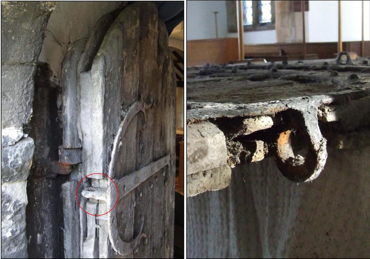
**Figure 1:** The Rainham hinge (left) and the Buttsbury hinge (right), showing similarities in their unusual formation.
